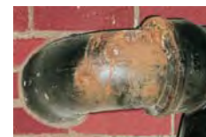
Prevention of corrosion and odour build-up
